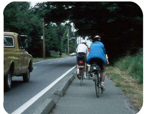
This is a barrier lane. Barriers can catch bicycle tires and inhibit the movement of cyclists.
