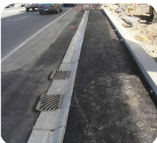
The bike lanes slope toward the center of the road for drainage. This means catch basins must be relocated to the mountable curb between the raised bike/parking lane and the motor vehicle travel lane.
