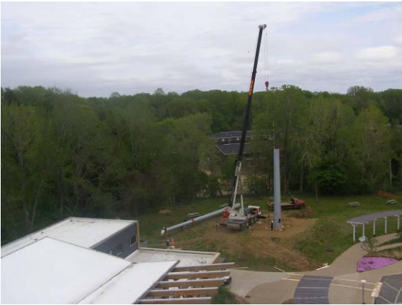
Fig. 2 The tower under constuction May 5, 2007
