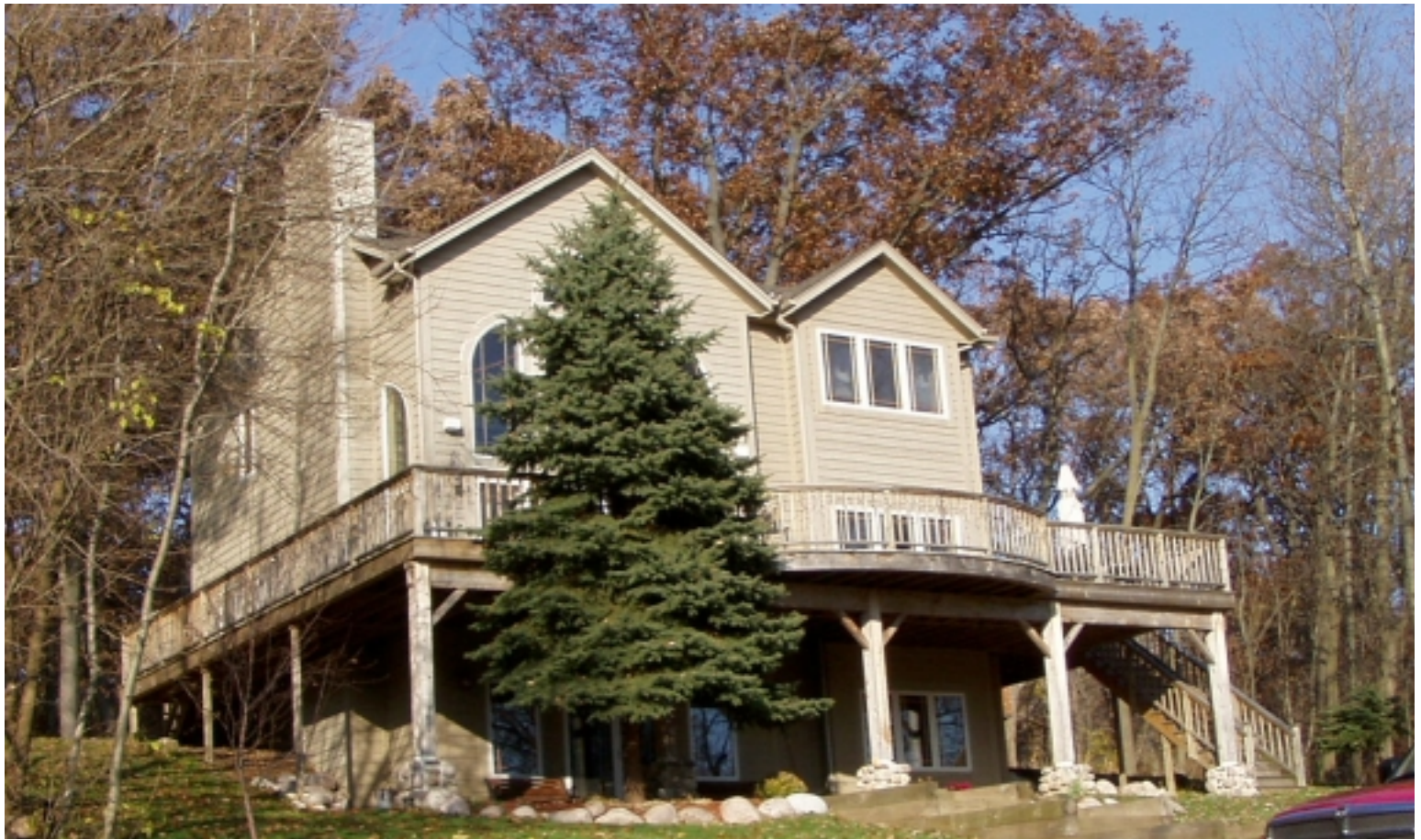
Warren S. Hornik's Home N27 W 300024 Maple Ave. Pewaukee, WI 53072
