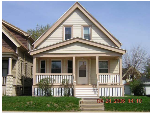
3226 North 35 th Street West End Development Corporation After
