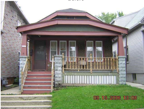
1317 West Scott Street Social Development Commission Before
