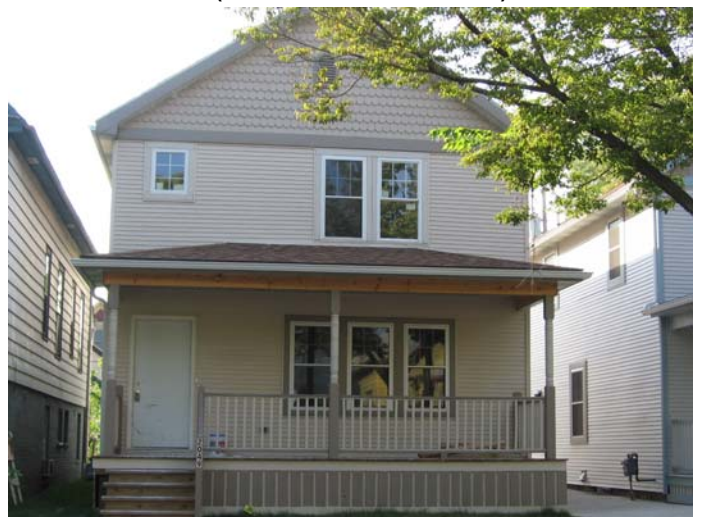
NEW CONSTRUCTION – FRESH START 2049 S. 15 th Street (Milwaukee Christian Center)
