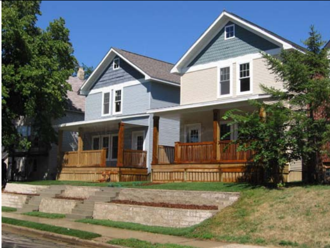
NEW CONSTRUCTION – CHDO 2324 & 2328 S. 16 th Street-(Milwaukee Christian Center)
