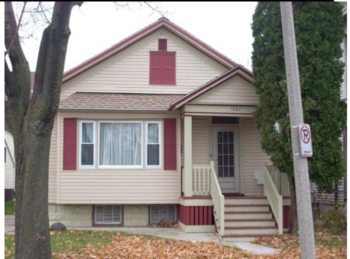
1227 South 10 th Street Milwaukee Christian Center After
