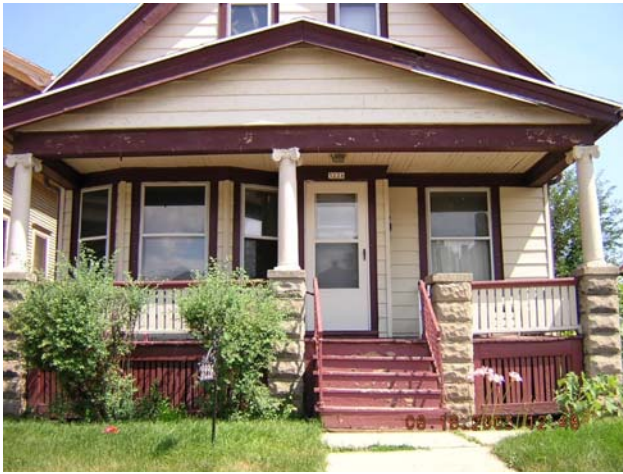
3226 North 35 th Street West End Development Corporation Before
