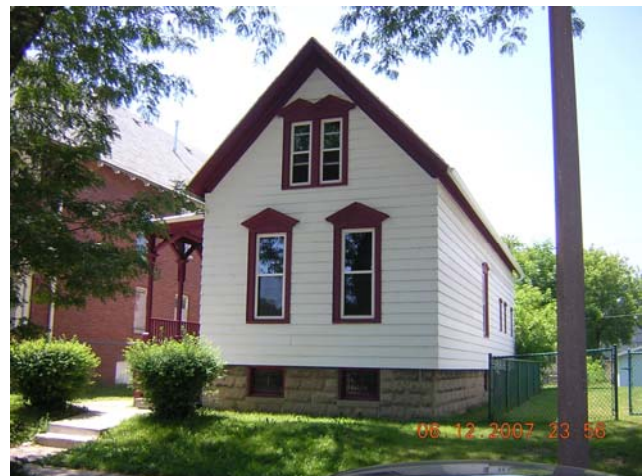
2935 North 4 th Street YMCA-CDC After
