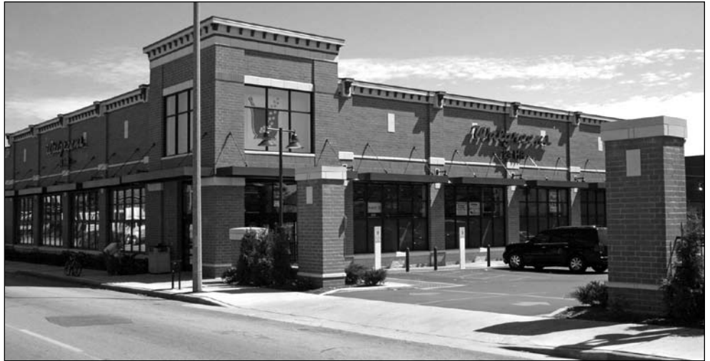
The new Walgreens is operating at S. 27th St. and W. National Ave. The store opened in June on the site where the National Liquor Bar and other businesses were located. Walgreens and the Redmond Company worked closely with the city and Ald. Donovan and the result is an important addition to the revitalization of the busy intersection.
