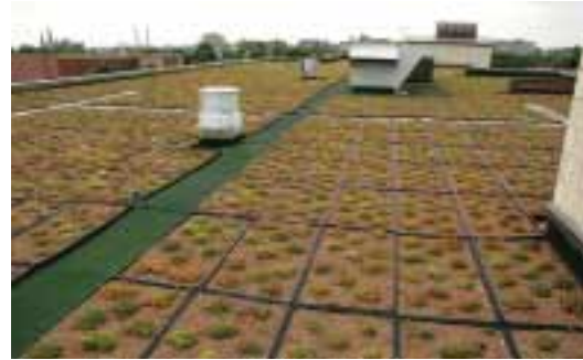
Figure 1: Highland Gardens Green Roof
