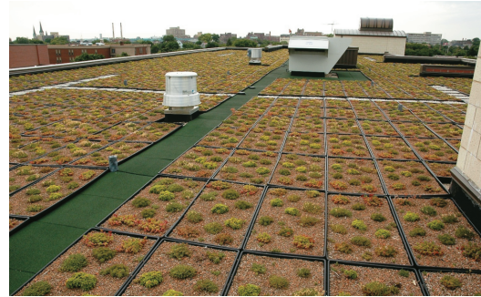
Figure 1: Highland Gardens Green Roof
