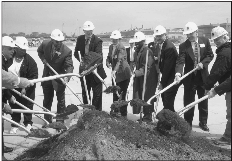
Participating in the groundbreaking for the new Department of Public Works/Milwaukee Water Works Maintenance Facility groundbreaking were (left to right) Sam Dickman Sr., The Dickman Company, Mrs. Wade (Alderman Wade's mother), Alderman Willie Wade, Mayor Tom Barrett, Superintendent of Water Works Carrie Lewis, State Representative Barbara Toles, Director of Operations Jim Purko, City Engineer Jeff Polenske, and Gerry Blomerg, Midwest Rail and Dismantling. Not pictured, State Senator G. Spencer Cogs, and Brian Byrne, president of Briohn Development.
